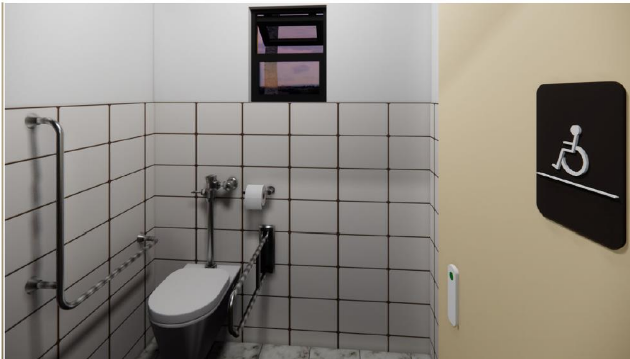
PHYSICALLY CHALLENGED – GRAB RAILS, WC, FLUSH VALVE AND TISSUE HOLDER
